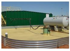
The earthen berm was removed and the site was graded for drainage. A gravity drain system was installed to handle precipitation. A 25-inch steel curtain berm was erected and a two-part elastomeric polyurea was spray applied to serve as secondary containment.
